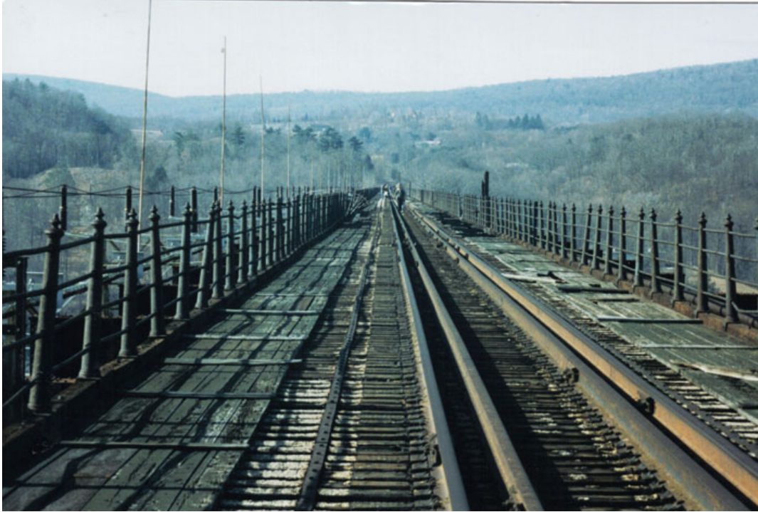
Fig 34. Decking, railings, and rail ties of the Poughkeepsie-Highland Railroad Bridge. Picture is taken looking west towards Highlands. Image accessed from http://walkwaypprd.marist.edu/historical-photos
