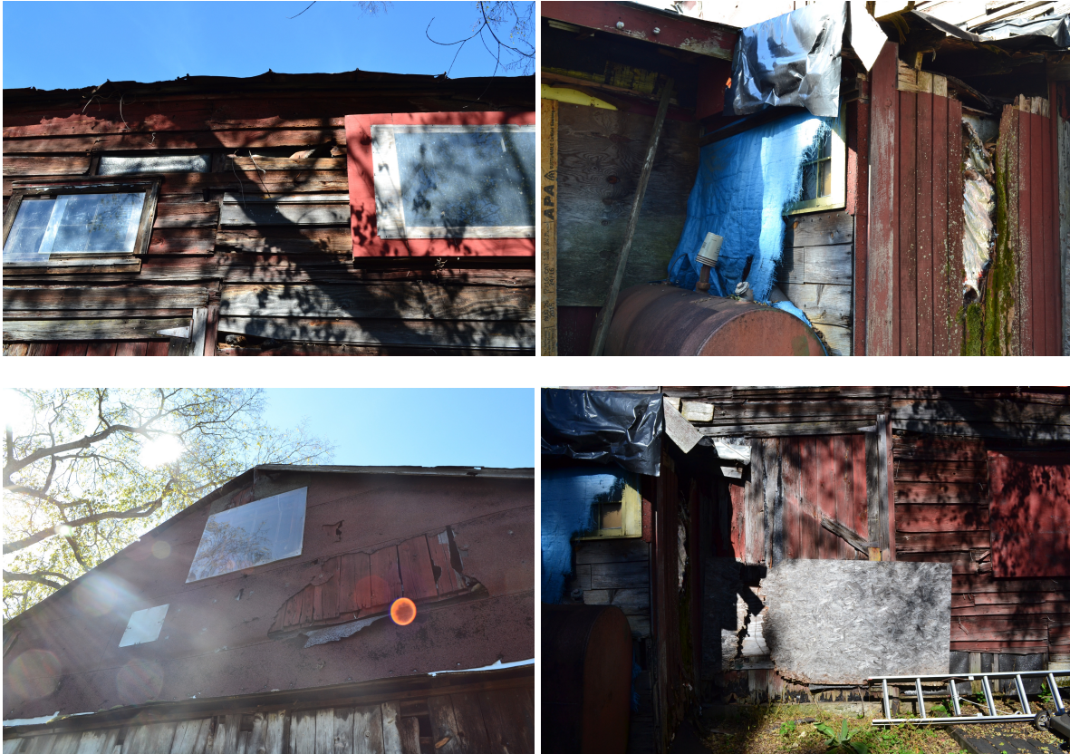
Fig 32. Four different images showing the exterior envelope condition on the rear façade of the Mill. All images taken by author.
