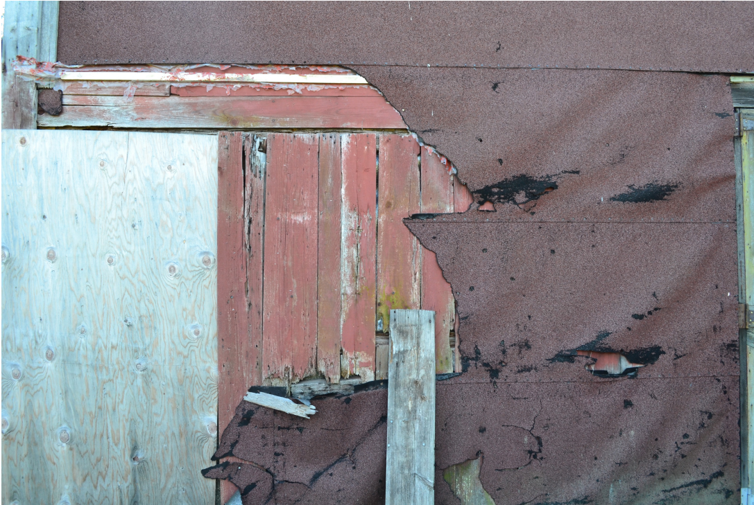
Fig 15. Plywood and tar paper cover the exterior of the rear addition. Image taken by author.
