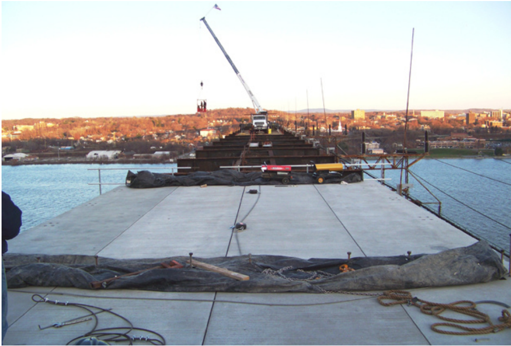
Fig 36. Pre-cast concrete decking being laid. Image taken looking east towards Poughkeepsie. Photo courtesy of the Walkway Over the Hudson Website, http://walkway.org/visit/visitor-photos/
