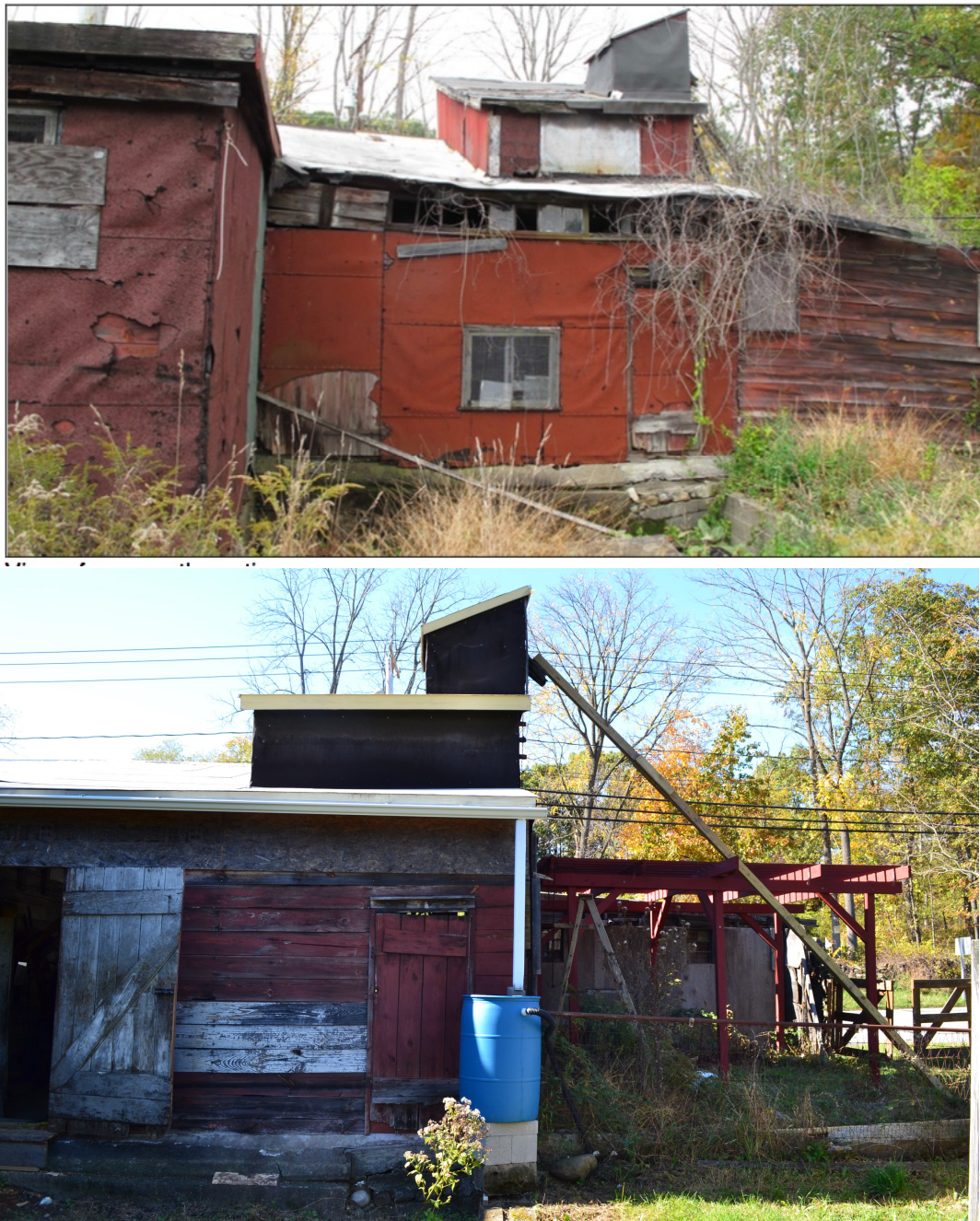
Fig 29. Before and after images of the Cider Press Room and roof dormer. In the bottom image, the dormer has undergone stabilization and repair. On the right of the image, a red, wooden pergola denotes the location of the north addition. Bottom image is taken from the east side of the building by the author. Top image taken from the Kimlin Cider Mill Existing Conditions Report, Selected Illustrations-3.
