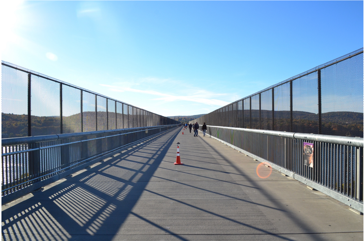
Fig 19. The precast, reinforced, concrete decking. Note the black chain link fence that occurs along portions of the walkway. Image taken by author.
