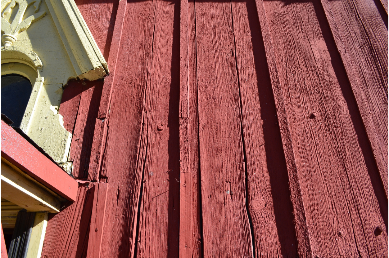
Fig 13. Close up of the vertical board and batten siding. Image taken by author.
