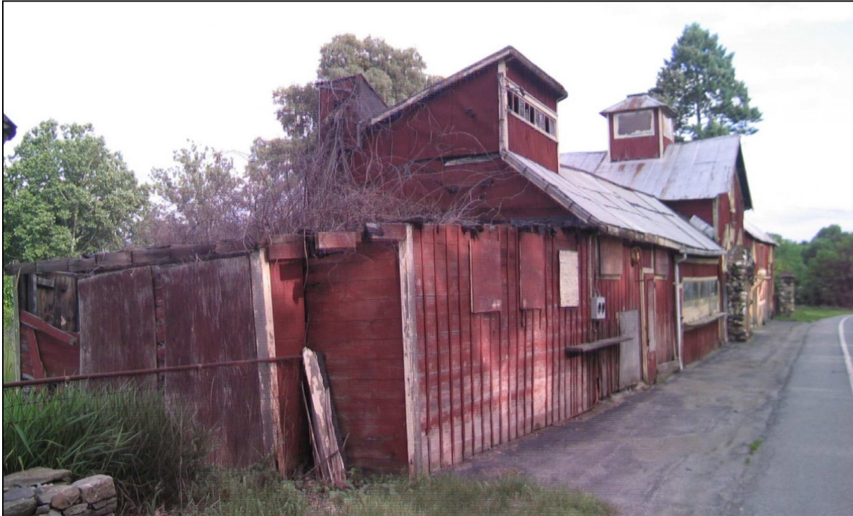
Fig 30. East and North facades of the small north addition. Note the sloping north wall and vegetation coming through the area of the roof. The east wall remains in fair condition. Image taken from Kimlin Cider Mill Existing Conditions Report, Selected Illustrations-2.
